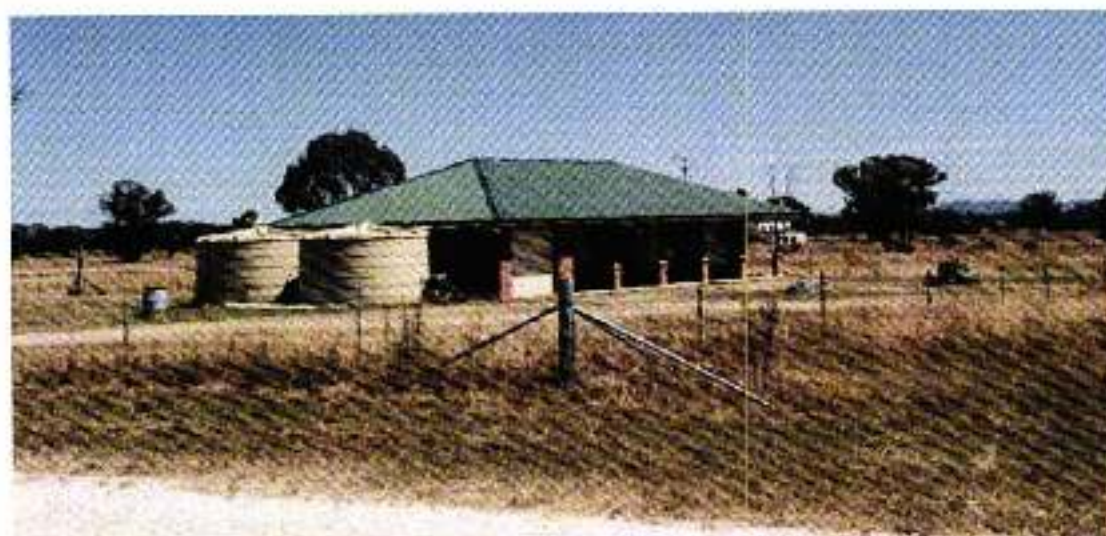
Photo 3: dual occupancy dwelling, looking south-west
